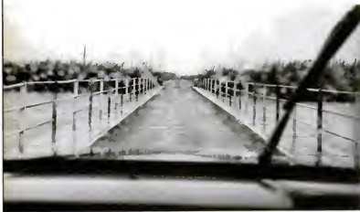
CHINESE PIPELINE. Unmanned Ruzizi River bridge (above) at Bujumbura leads into Congo and is used to smuggle arms to rebels. Two other bridges were blown up by Tshombe forces. Map shows route Chinese use
